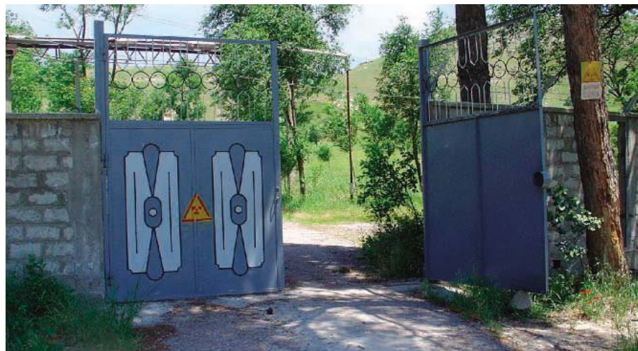
Isolation. Barriers have been upgraded at the Faizabad radwaste site, with help from the U.S. Department of Energy.
